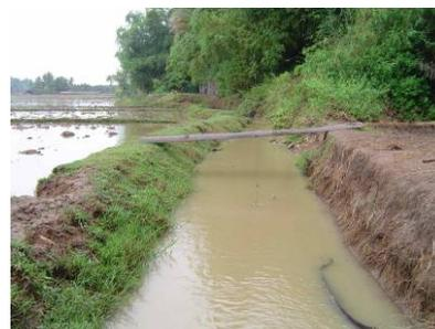
The irrigation schemes have an operational water supply system and some basic drainage channels – though what the farmers call drainage is really overflow systems that remove excess irrigation water from one irrigated field to the next field down-slope.
